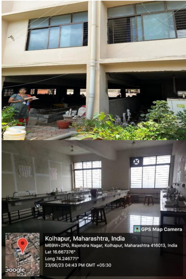
Fig. No. 10 Rain Water Recharging collection pipeline
