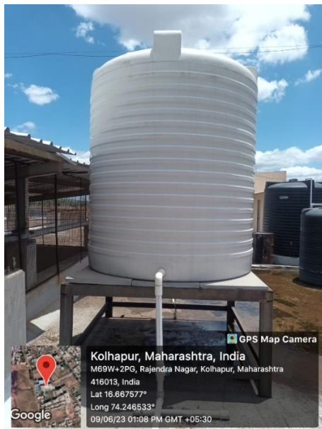
Fig. No. 5 Water Storage Tank at Terrace
